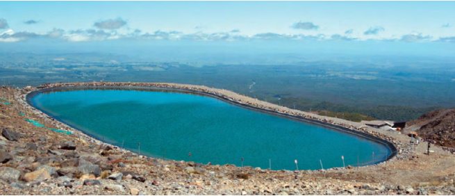
LDPE lined reservoir
